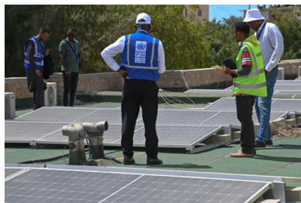
Training session with UNDP staff on solar system installation, Nouakchott, Mauritania. Photo: UNDP Mauritania
