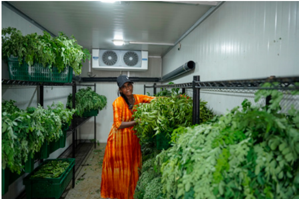
With a capacity to store up to 5,000 kg of vegetables, this solar-powered containerized cold room helps buy, store and sell the local vegetable production. Photo: UNDP Sri Lanka
