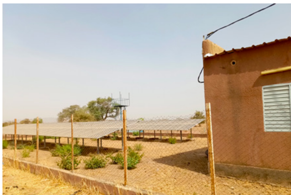
Solar minigrid installation in rural Nigeria.
