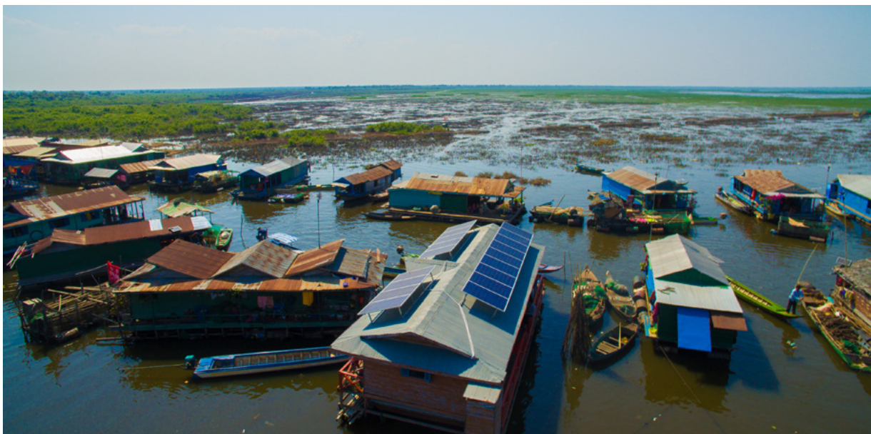
Floating community in Cambodia with on roof solar panels. Photo: UNDP Cambodia
