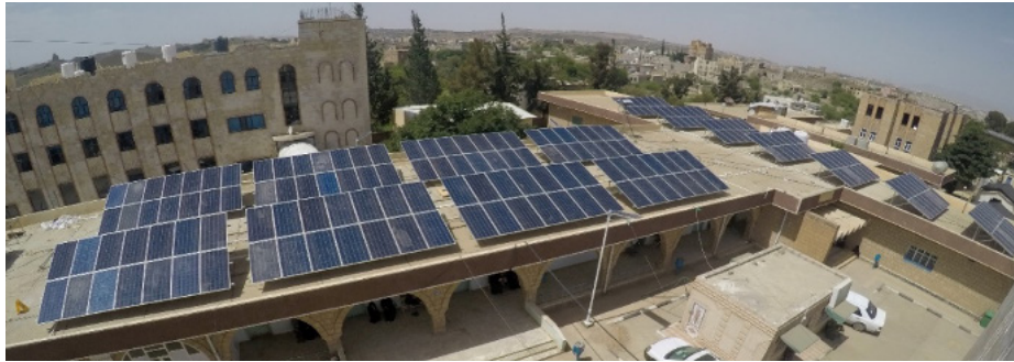
With an installed capacity of 110 kWp , the photovoltaic energy installation in UNDP's Sanaa office is the largest solar energy installation in the Arab States region. Photo: UNDP Yemen
