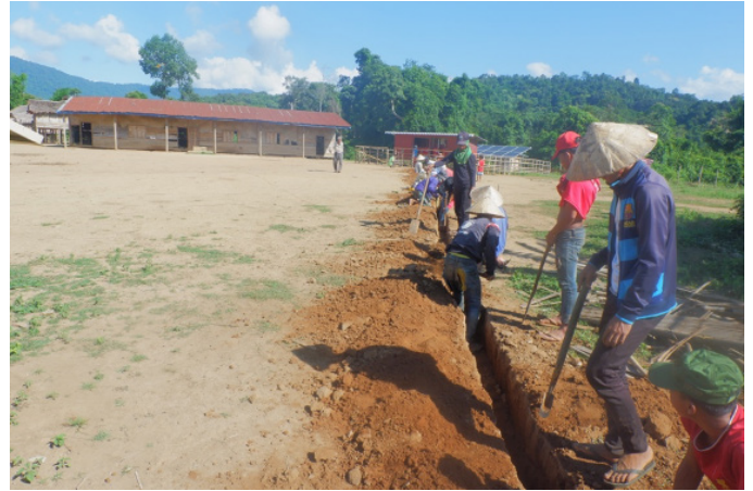
Figure 11: Digging trenches for the mini-grid
