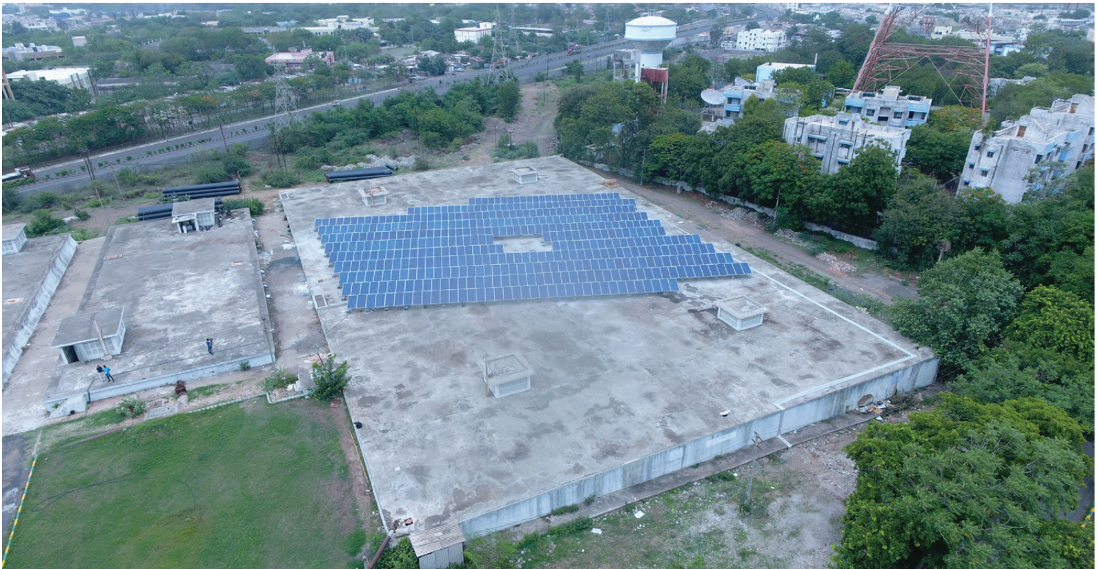
Rajkot, India, and Urban-LEDS project city, has installed a 145kWp solar PV system to help power its Aji water treatment plant
