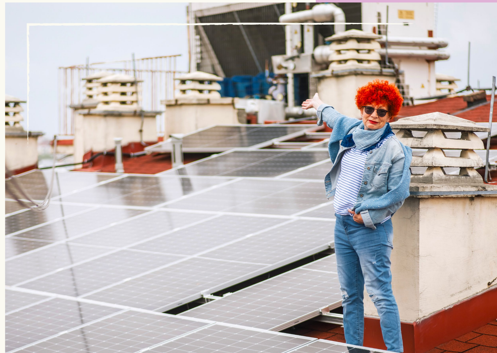
With a passion for community and the environment, Vesna led the 134 apartments in her building complex to invest in the installation of solar panels. © UNDP Serbia
